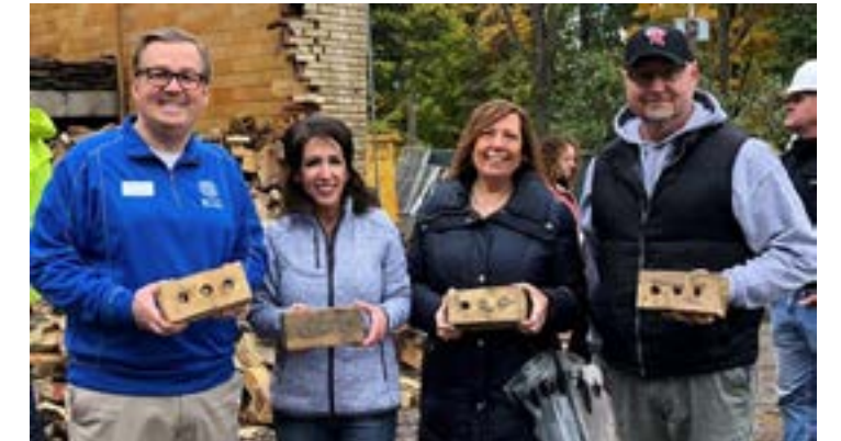
Larry, Cheryl, Pamela Reed Sanchez (President and CEO of Seneca Park Zoo Society), and Richard Mikiciuk (Assistant Zoo Director – Facilities) participated in the Main Zoo Building Demolition Ceremony... and they have the bricks to prove it.
